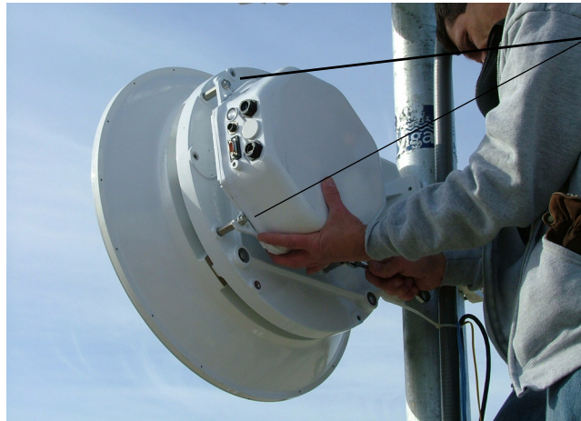
Tightening Radio Head Mounting Bolts
