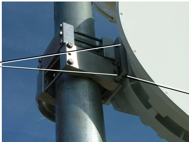
U-clamp over Mounting Assembly Collar
